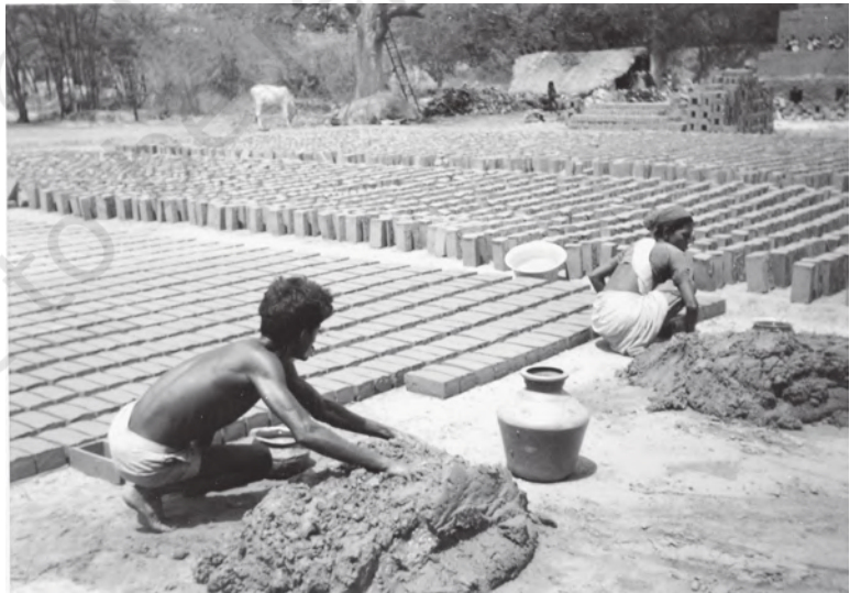
Fig. 7.2 Brick-making: a form of casual work
