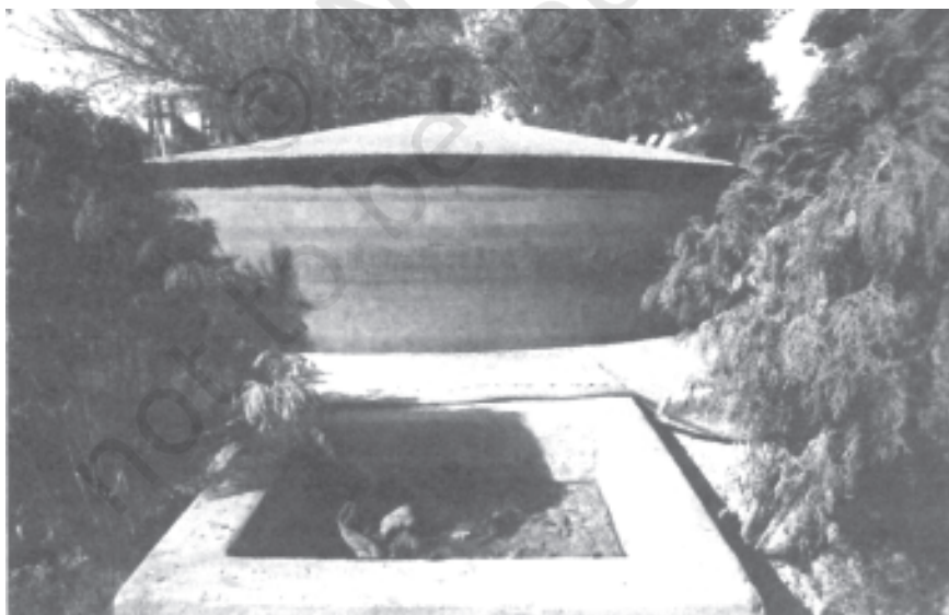
Fig.9.4 Gobar Gas Plant uses cattle dung to produce energy
