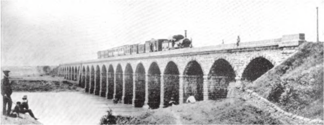
Fig. 1.4 First Railway Bridge linking Bombay with Thane, 1854
