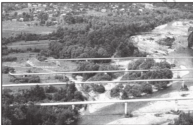
Fig. 8.17: Pipelines transporting natural gas in Ukraine
