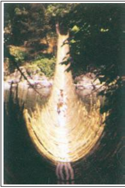
Figure 6.7 : Rope Bridge (Arunachal Pradesh)
