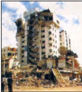
Fig. 3.3a: Destruction caused by an Earthquake in Gujarat
