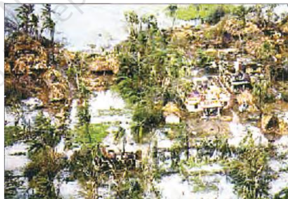
Destruction caused by a cyclone
