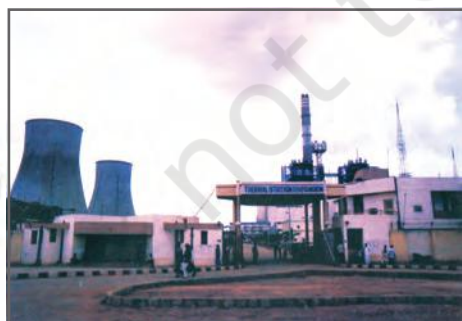
Fig 3.10: A view of a Thermal Power Station
