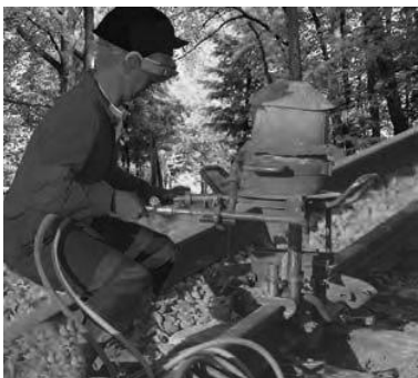
Figure 3.11 Thermit process for joining railway tracks
