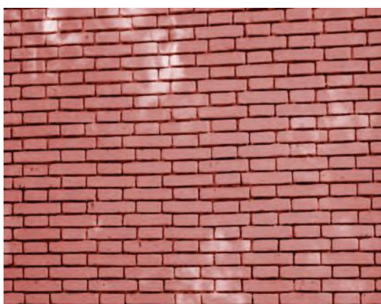
(a) Brick wall
