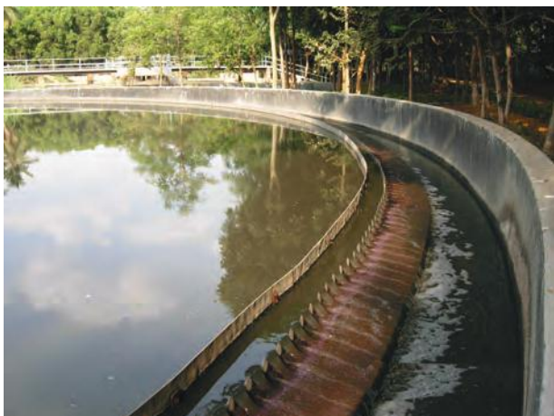
Fig. 18.5 Water clarifier
